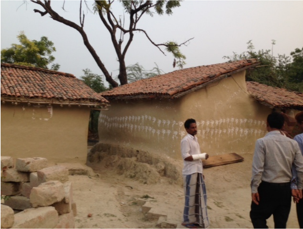
Image 1: Houses with tile roof, mud walls and mud floor
