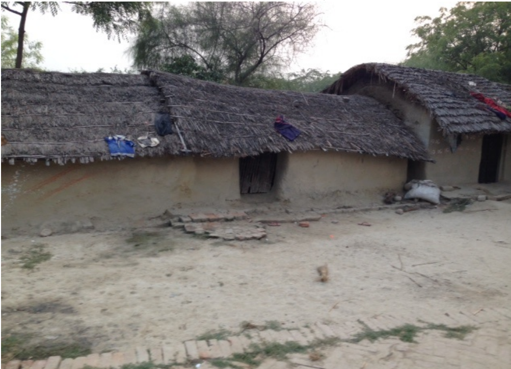
Image 2: House with thatched roof, mud walls and mud floor
