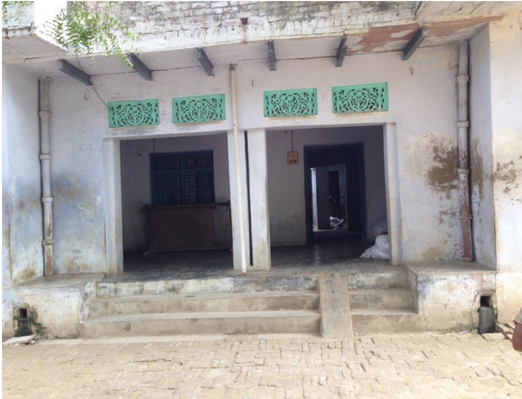
Image 3: A better house with cemented floor, plastered walls & reinforced cement roof
