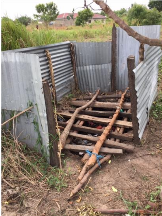
Poor quality pit latrine
