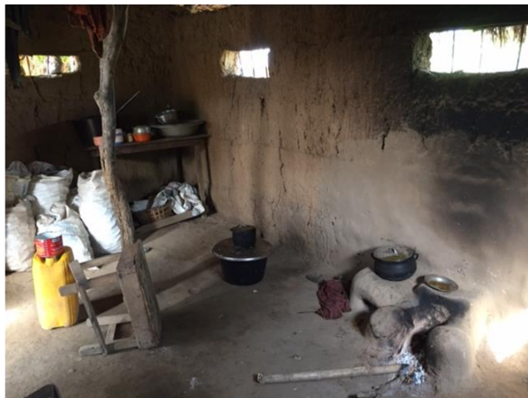
Cooking area with inadequate ventilation
