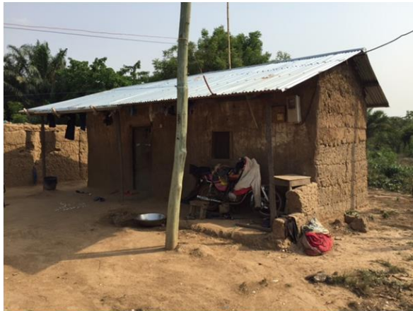
House with mud brick walls
