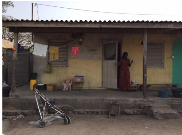
Good construction but insufficient space
